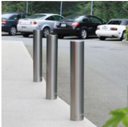
Bollards Pedestrian Safety
